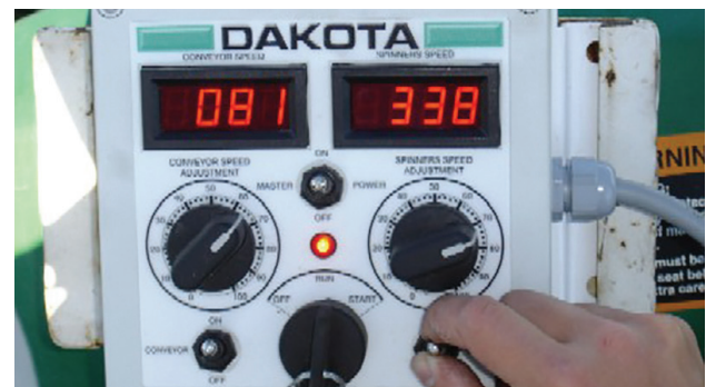
Electric Control Box
